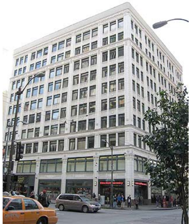
Image courtesy Joshua Green Corp. and Artifacts The L-shaped building at Fourth and Pike was constructed for tenants that wanted 500 to 2,000 square feet. The goal is to attract tenants needing 6,000 to 10,000 square feet.
